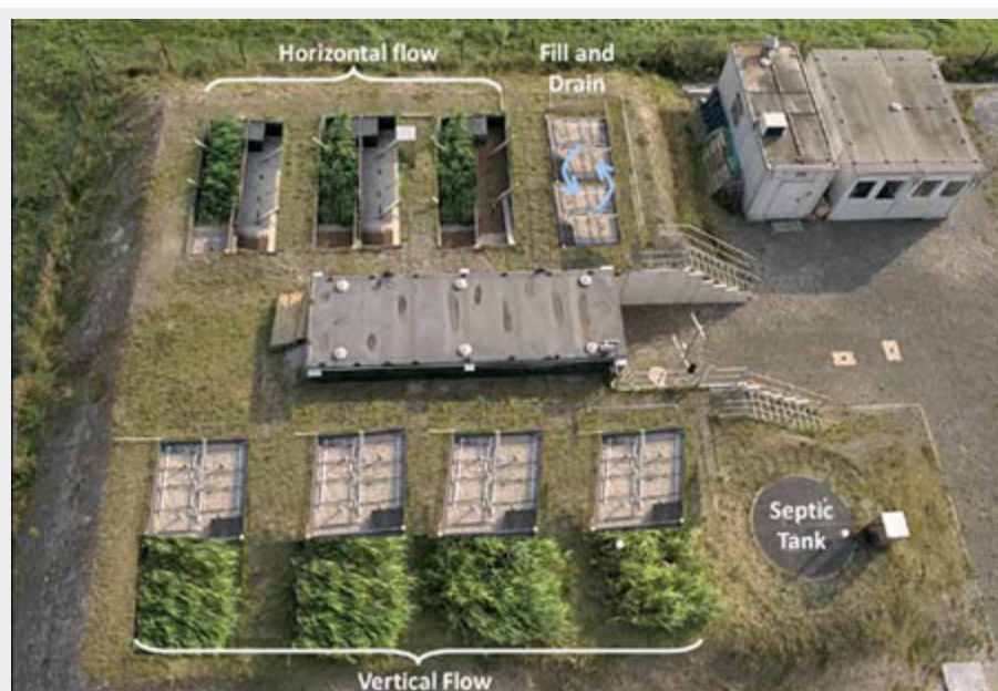
The Langenreichenbach research facility contains 15 standalone treatment wetlands of seven different designs.
